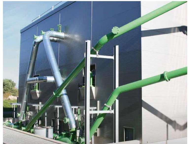
Discharge system of a Kompogas® concrete digester
