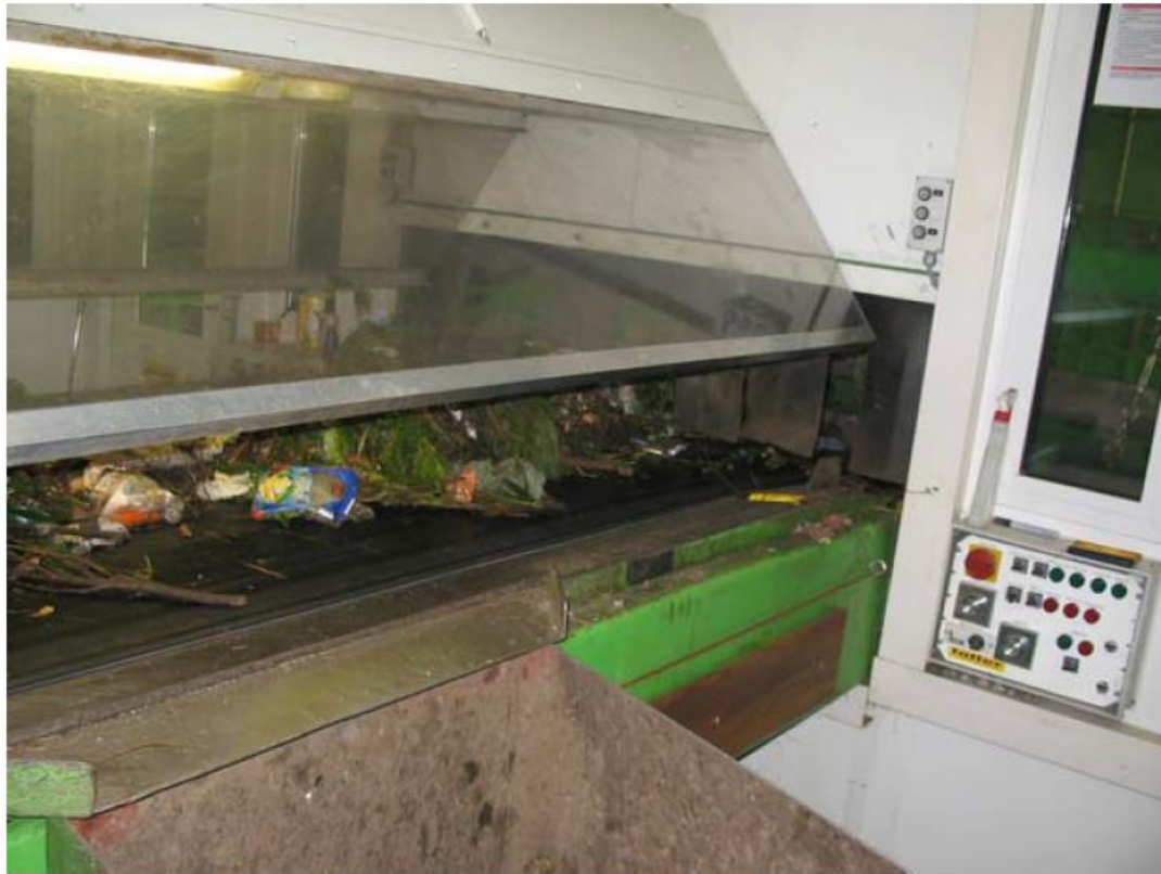
Figure 3-2: Contaminant removal (sorting) station.
